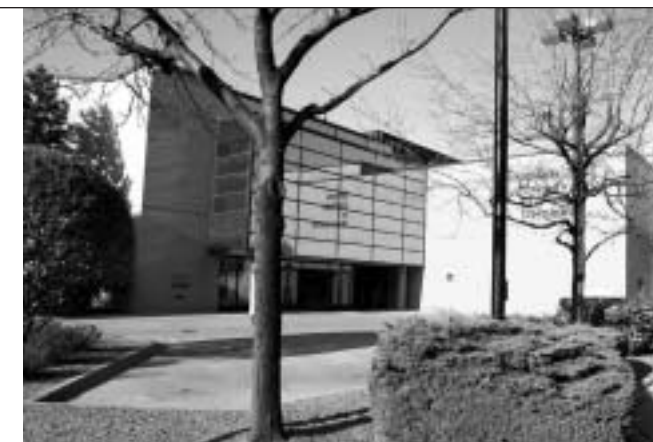
The entrance to the Illinois College of Optometry, Indiana Avenue, between 32nd and 33rd streets
